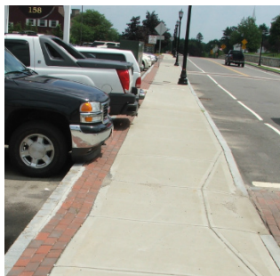
Most of the sidewalks in the town center have smooth surfaces.
