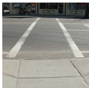
Crosswalk with curb cut ramp
