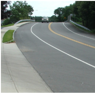
The shoulders along Main Street are wide enough to fully accommodate bicyclists.
