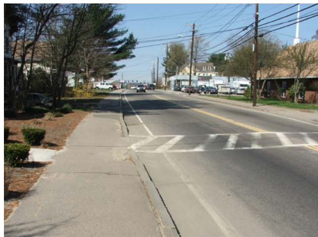
Plymouth Street, looking west
