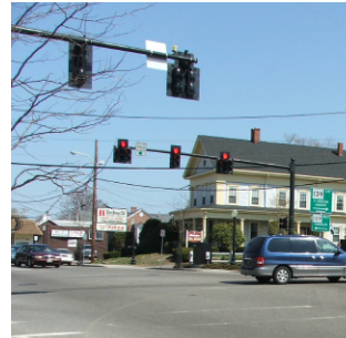
This intersection was reconstructed in 2002.
