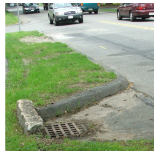
Drainage grates are set back from the roadway.
