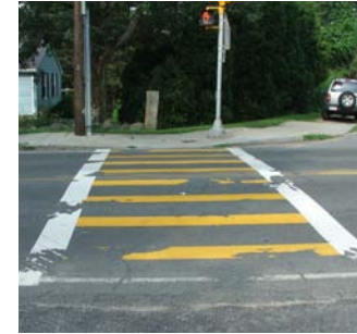
Signalized pedestrian crosswalk across Marlboro Road
