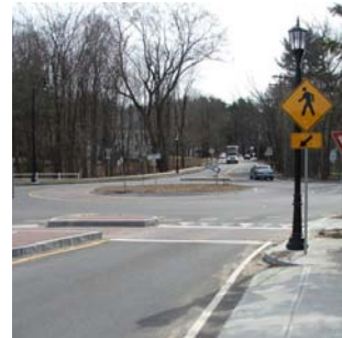
Two roundabouts were recently installed in the town center.
