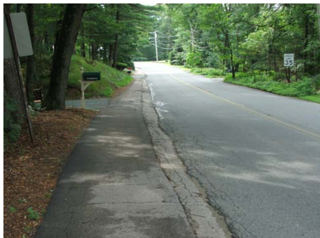
North Street, looking southeast
