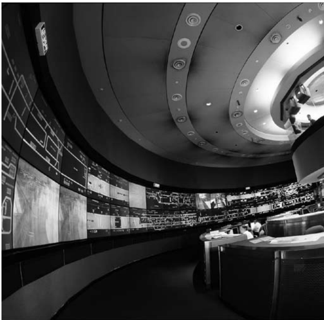
MBTA SUBWAY OPERATIONS CONTROL CENTER
