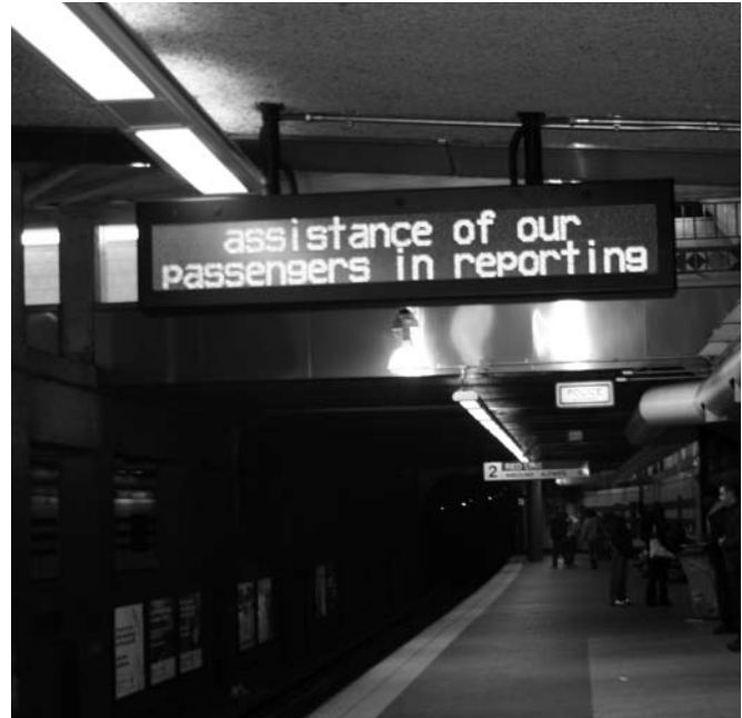
VARIABLE-MESSAGE SIGN IN MBTA STATION
