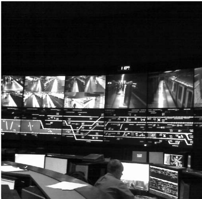
MBTA OPERATIONS CONTROL CENTER – CCTV UPGRADE
