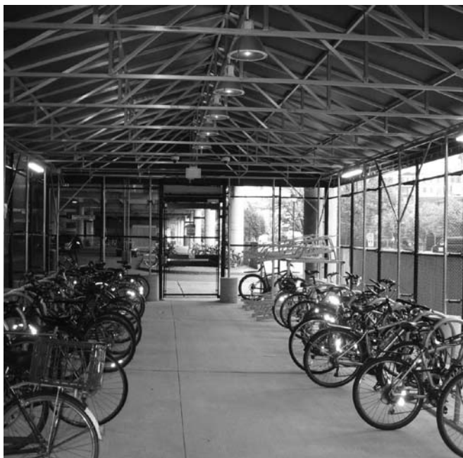
MBTA BIKE CAGE FACILITY
