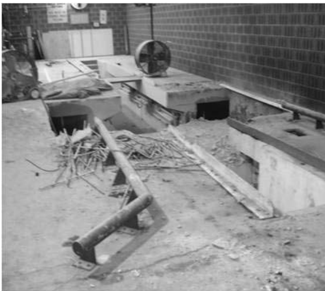
EVERETT MAINTENANCE FACILITY RECONSTRUCTION
