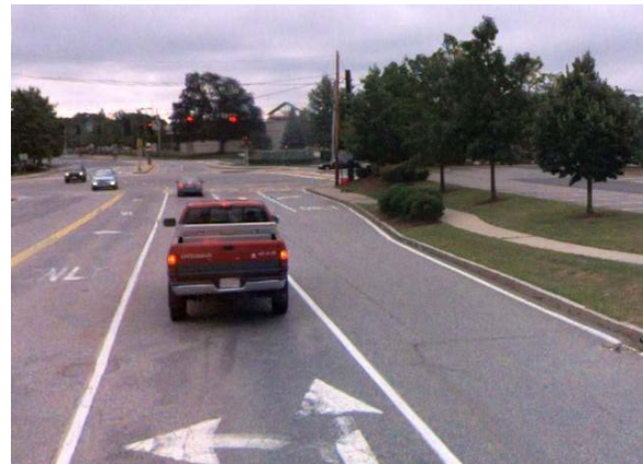
Sidewalk with grass buffer on Whittier Street
