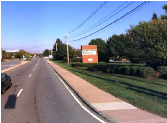
Sidewalk without a buffer on Route 30
