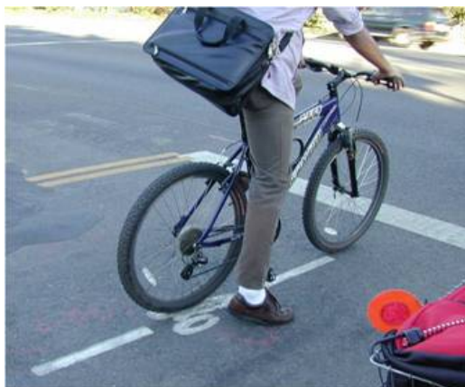
Bicycle detector pavement marking
