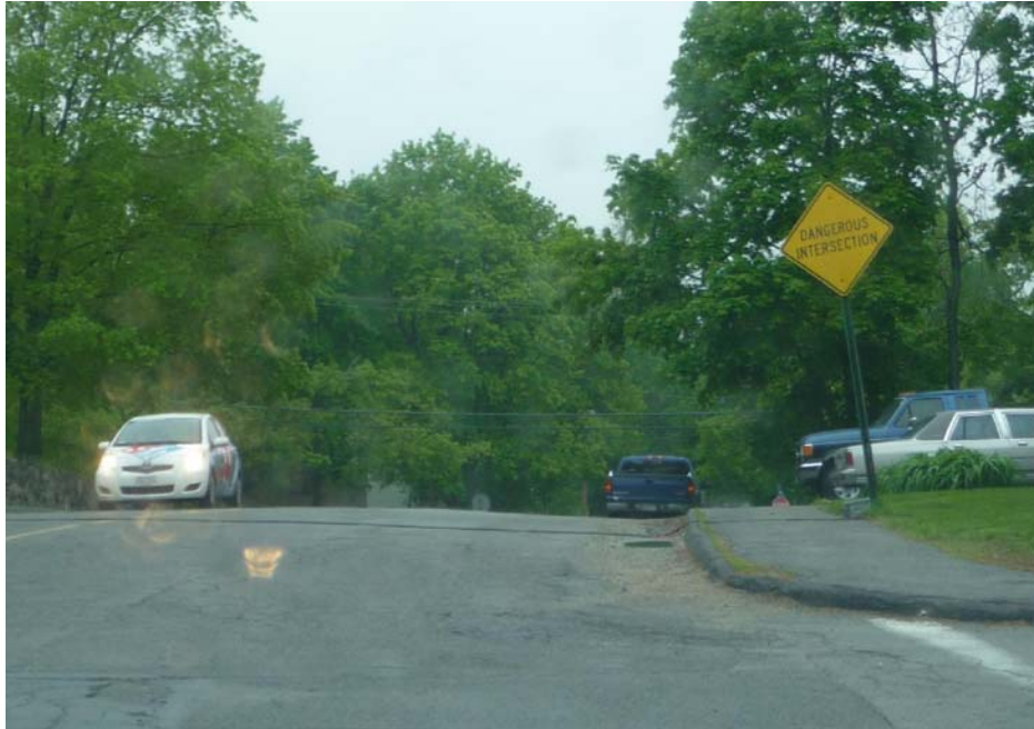
FIGURE 3 “Dangerous Intersection” Sign on Packard Street
