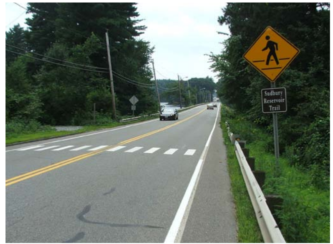
Cordaville Road, looking south
