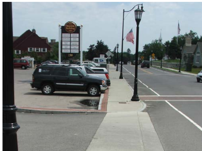
Main Street, looking east
