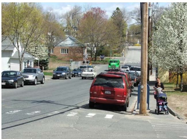
Main Street, looking east
