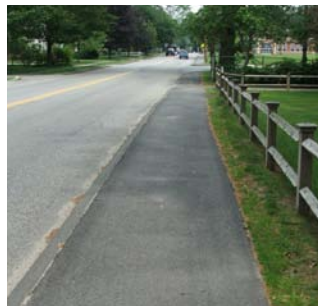
Lynnfield Center has a comprehensive sidewalk network.
