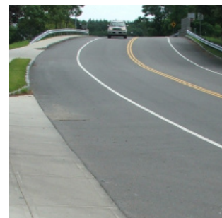
Smooth roadway surface
