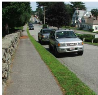
Sidewalk with a buffer
