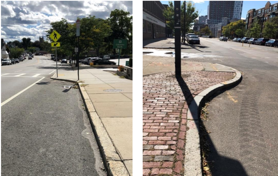
Curb extensions crossing Centre Street (left) and Tremont Street (right) in Boston, Massachusetts.
