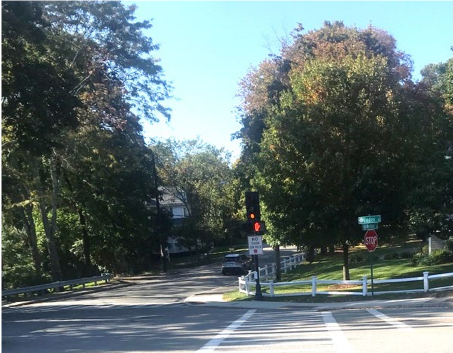
Figure 9 View of North Corner Curb Ramp and Detectable Warning Strip Pairs
