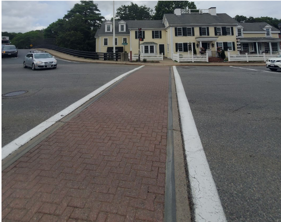
Figure 11: Long crosswalk with limited high visibility marking.
