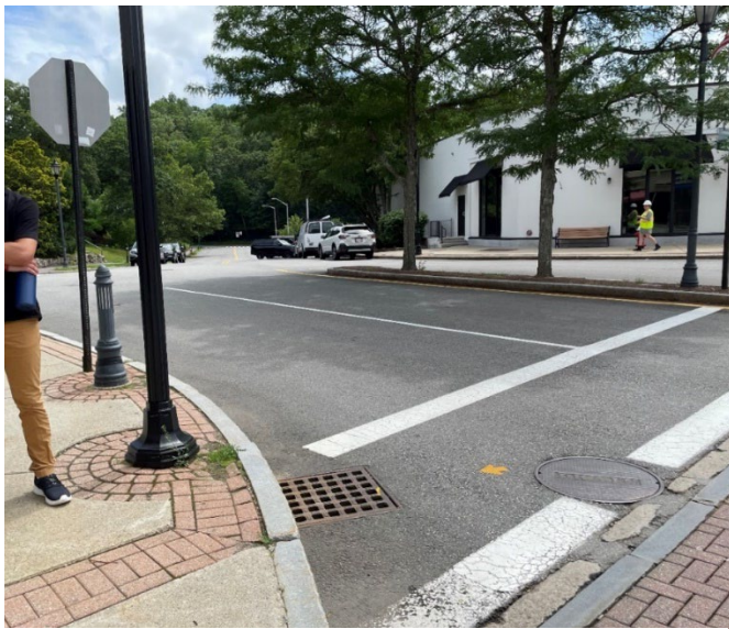
Figure 15: Stop sign set back from stop bar on the Cross Street approach to Central Street
