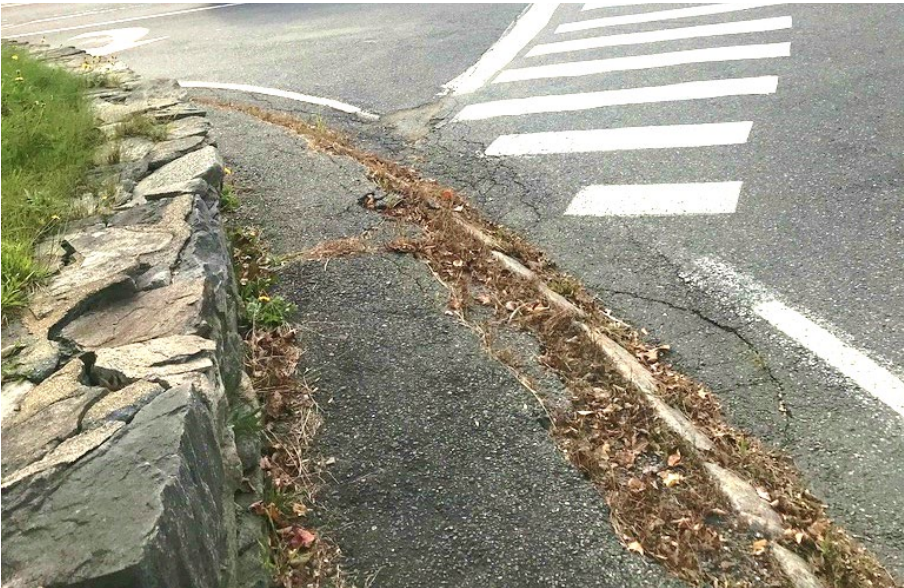
Figure 16 Southeast Intersection Corner Crosswalk Lacking Pedestrian Facilities
