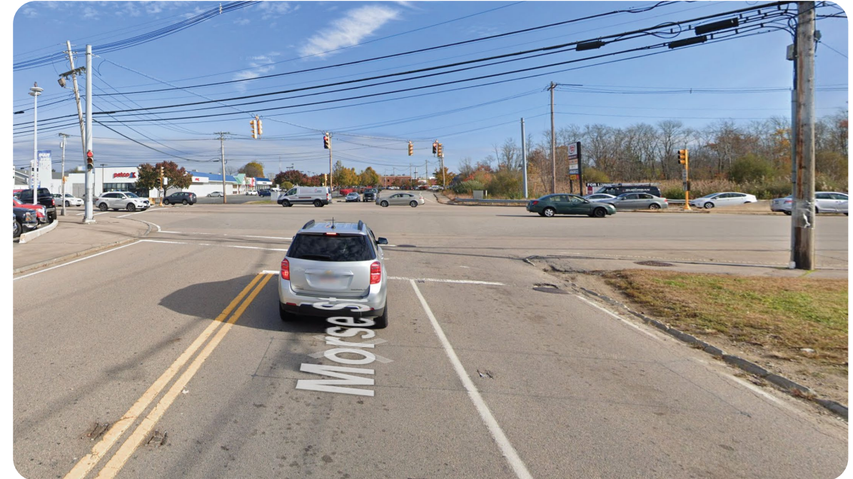
Lack of pedestrian signals and pushbuttons on Morse Street
