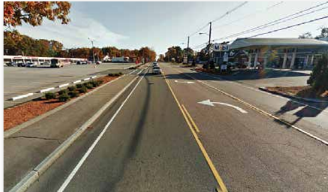
Route 109 in Medway Two-lane, two-way roadway with a two-way left-turn lane and sidewalks
