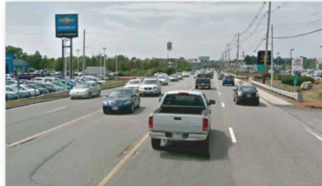
Route 114 in Danvers Four-lane, two-way roadway with a two-way left-turn lane and sidewalks
