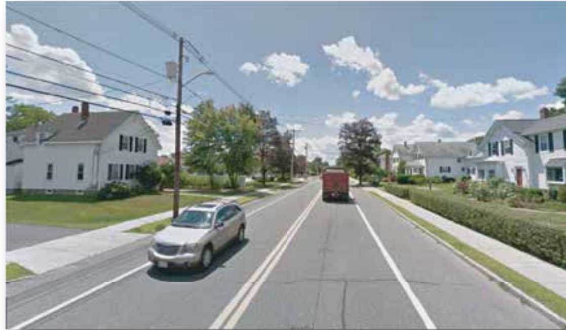
Route 135 in Natick Two-lane, two-way roadway with shoulders and sidewalks with buffers
