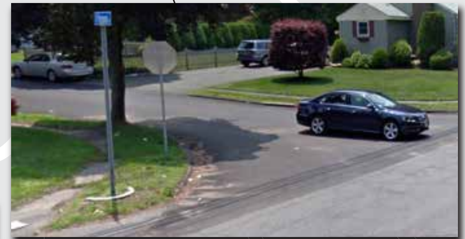
Poor sidewalk and need for crosswalk
