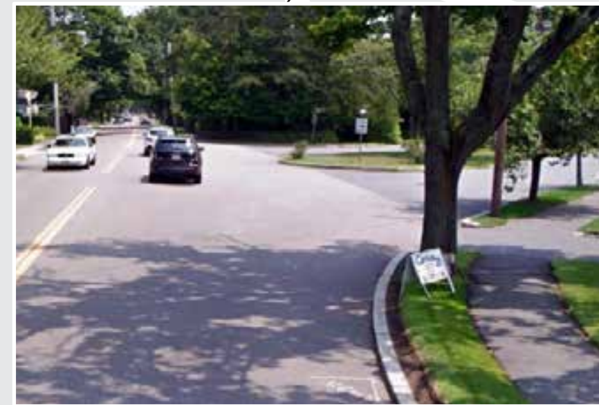
Lack of crosswalk and long and unsafe crossing distance
