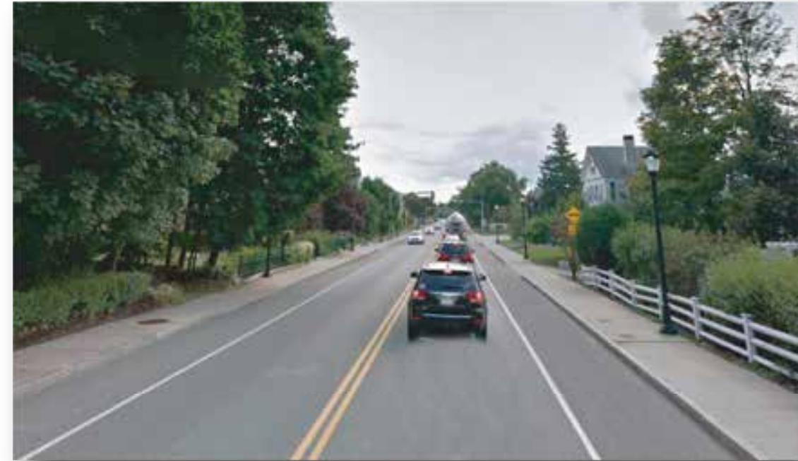
Route 109 in Westwood Two-lane, two-way roadway with shoulders and sidewalks
