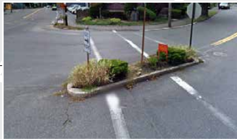
Obstruction in crosswalk (not ADA compliant)
