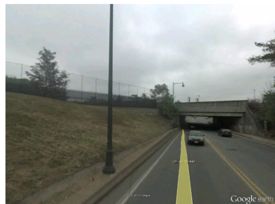
Union Street: location for north-side sidewalk and pedestrian bridge
