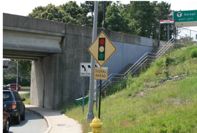
Access to the Braintree Station elevated pedestrian walkway
